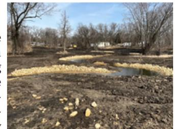
Figure 1 shows finished stream restoration section below culvert under Woodhaven Drive East looking at the area between sections 8 & 9.
